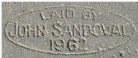
Concrete in sidewalk stamped with contractor name and date it was laid
