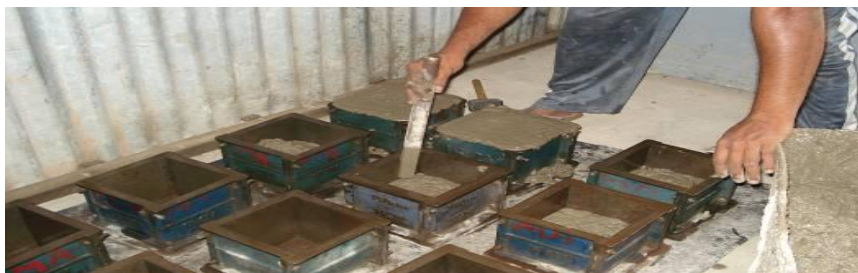
compacting of concrete cubes
