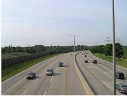
A highway paved with concrete.
